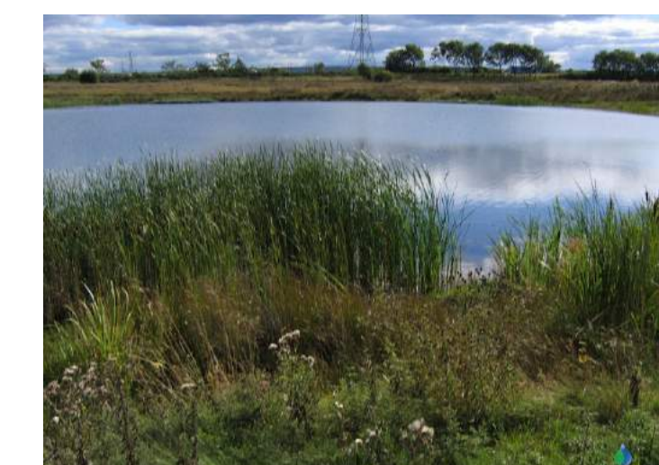
(5) Retention pond with added vegetation to encourage ecological growth
